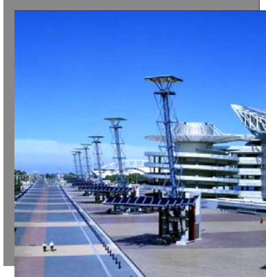
Figure 9: Photovoltaic towers for street lighting
